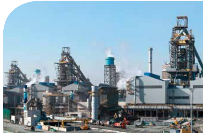
Paul Wurth supplied the engineering and key components for blast furnaces 1, 2, and 3 of Hyundai Steel, South Korea.
